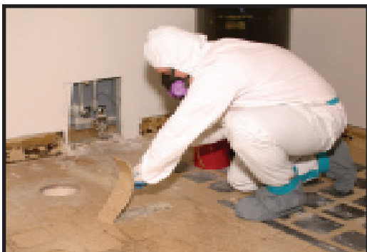
Prying up a section of flooring
